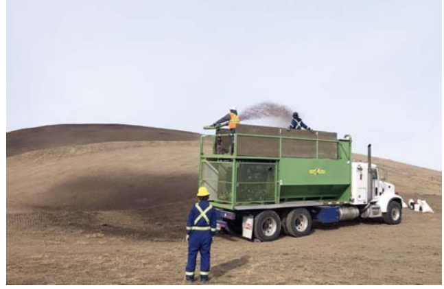
In some areas seed was applied wet, with a tackifier, to adhere to dry slopes.
