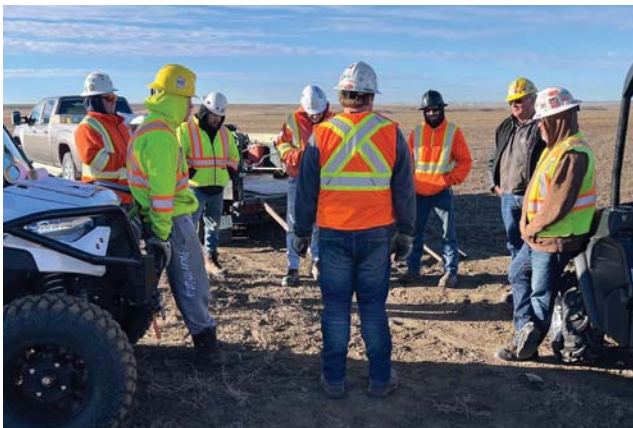
For the restoration crew, each morning began early with a "tailgate" safety meeting to discuss the day's work.
