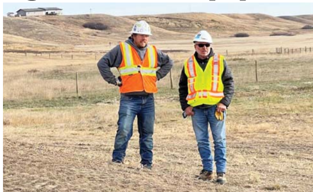
Line 3 Construction Manager Allen Sawatzky (right) and contractor Brodie Charteris checking progress along the RoW.
