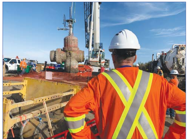
Above: A worker looks on during removal of a valve south of Morden.
