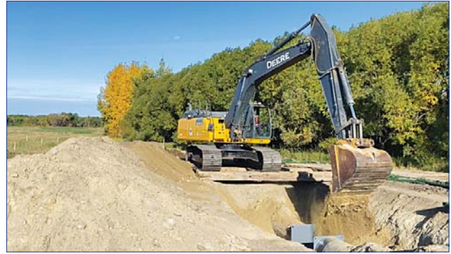
Above: Once the cap is in place, backfilling of the excavation begins.
