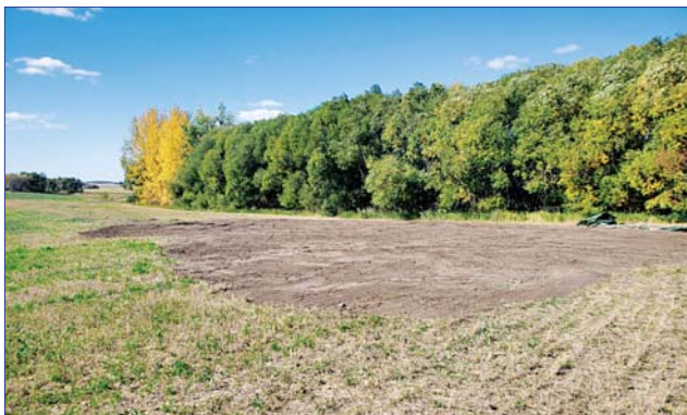
Above: With backfill completed and the topsoil replaced, the land is ready to be returned to its pre-construction state.
