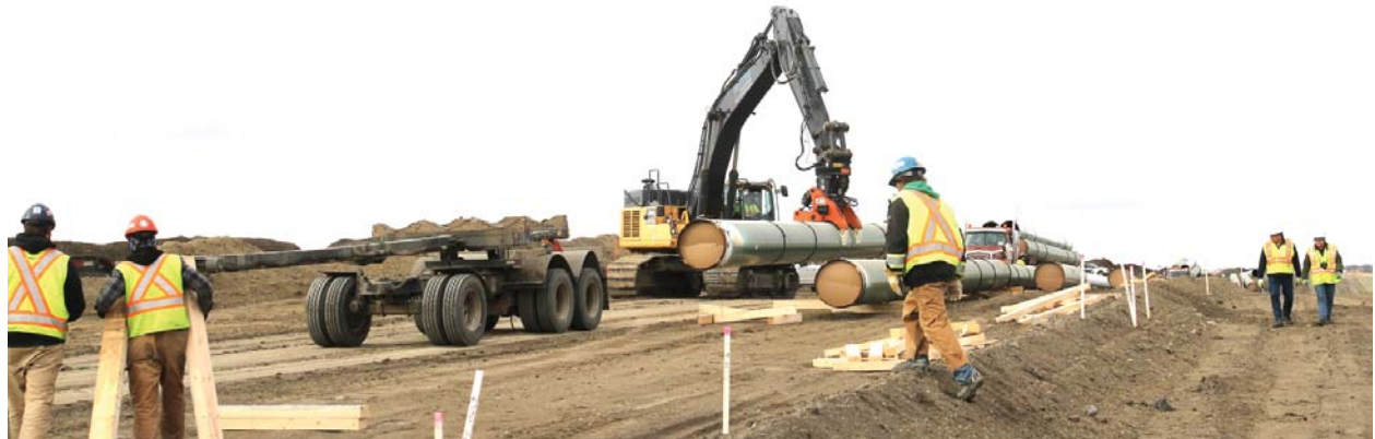
Pipe being unloaded along the right-of-way near Kipling. This crew was advancing at about 4.5 km per day, getting the pipe laid out.
