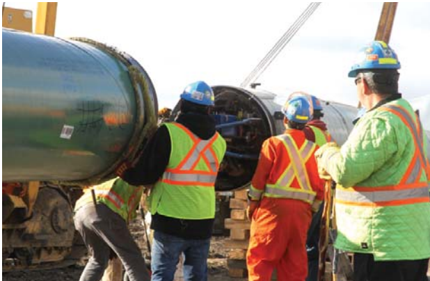
Above: Two joints of pipe come together before being welded.
