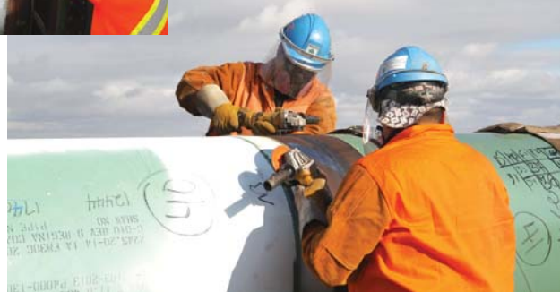
Right: Buffing one of the welds.
