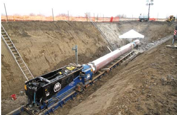
Track boring under the rail line between Fairlight and Maryfield.
