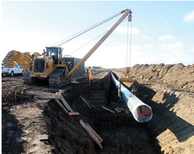
The pipe is laid into the trench.
