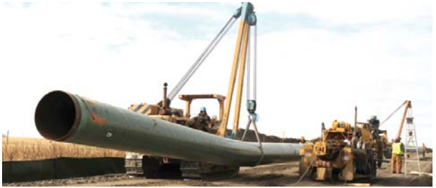
Pipe being unloaded along the right-of-way near Kipling. This crew was advancing at about 4.5 km per day, getting the pipe laid out.
