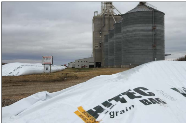
Parrish and Heimbecker has 24 grain bags at the Moosomin terminal. Each bag holds enough grain to fill three rail cars.
