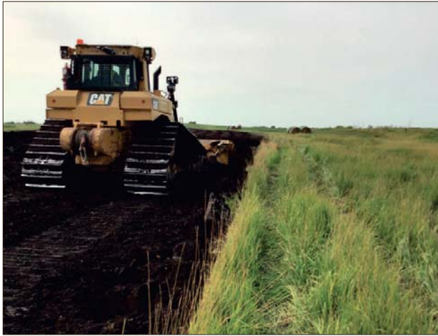
Left: Near Kelso, the last piece of land along the 1,070-km Line 3 replacement pipeline right of way has been reclaimed to pre-construction condition or better.
