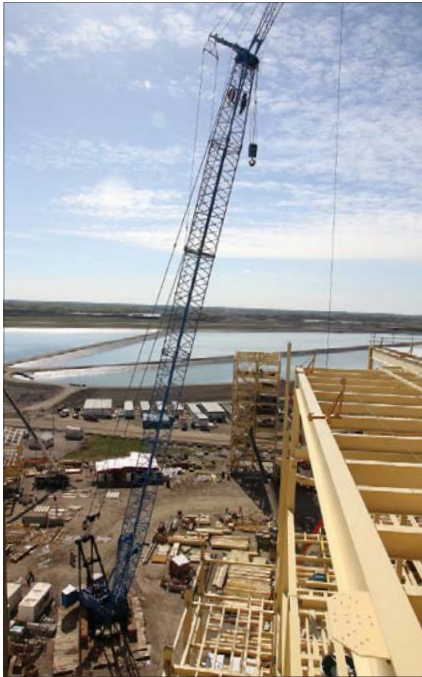
A crane works on adding sections to the new mill.
