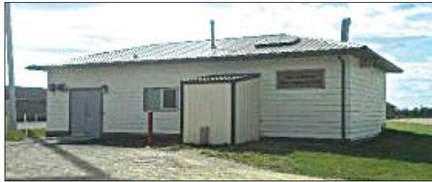
The current Redvers water treatment plant. An addition will be made to the existing plant to house the new water treatment infrastructure being done as part of a major water treatment upgrade.
