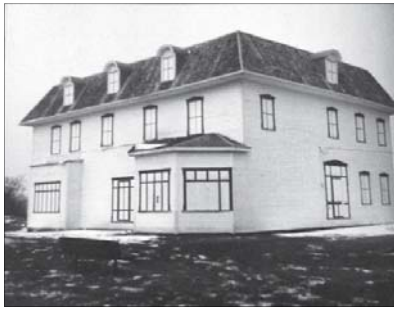
Above: A photo of the boarded up Humphrys-Hewlett house at Cannington Manor.
