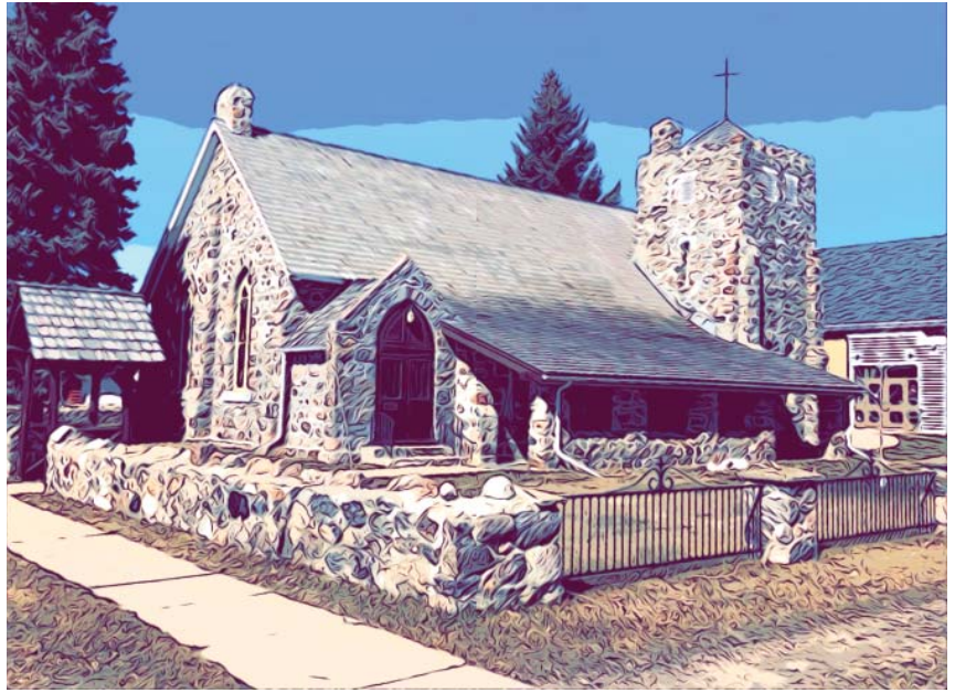
St Mary's Anglican Church in Virden is a unique example of fieldstone construction.
