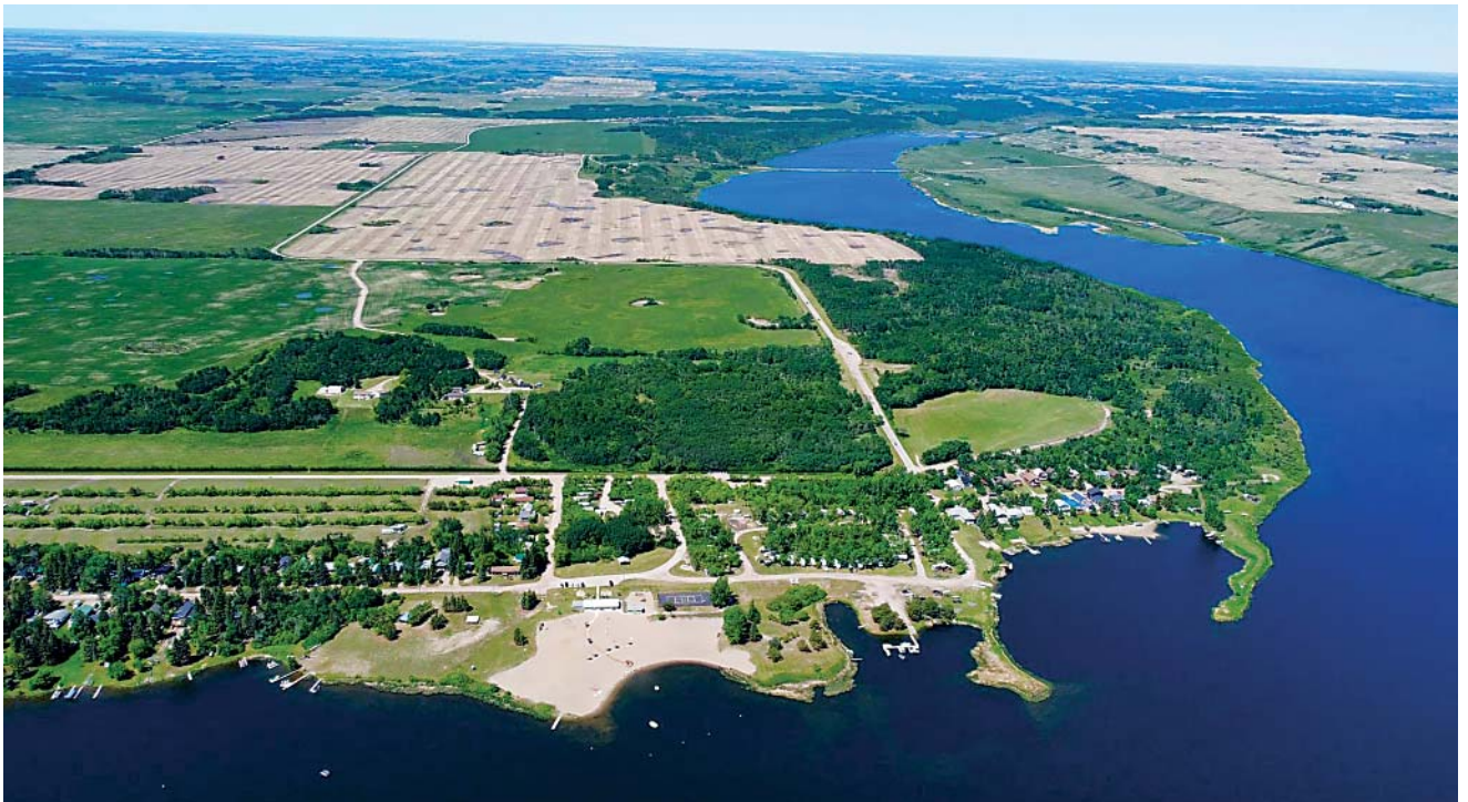
Above: An aerial view showing the beach and Moosomin Lake over to the dam.
