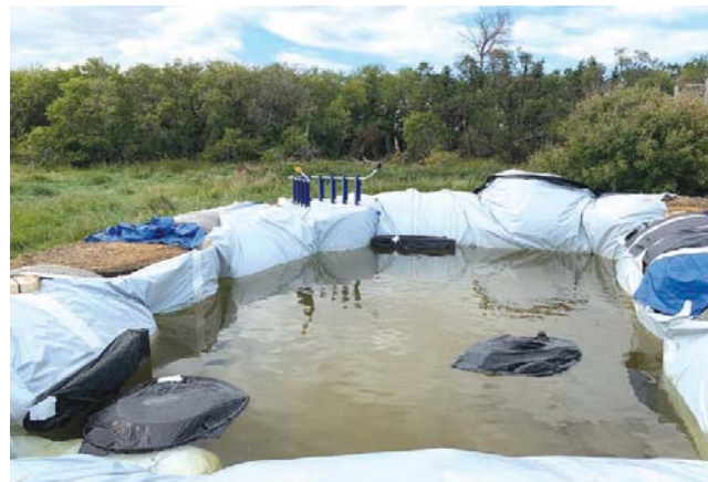
Hailey Gibson wanted a pool, so she decided to build her own using hay bales and plastic tarps. To keep it heated she built her own solar heaters from pool noodles and hula hoops (the black objects in the bottom right photo).
