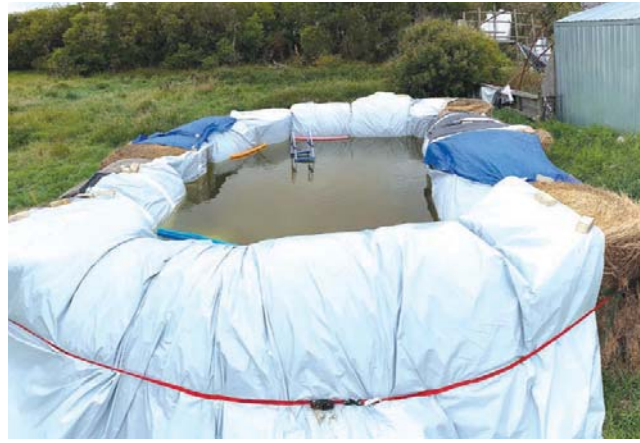
Hailey Gibson wanted a pool, so she decided to build her own using hay bales and plastic tarps. To keep it heated she built her own solar heaters from pool noodles and hula hoops (the black objects in the bottom right photo).
