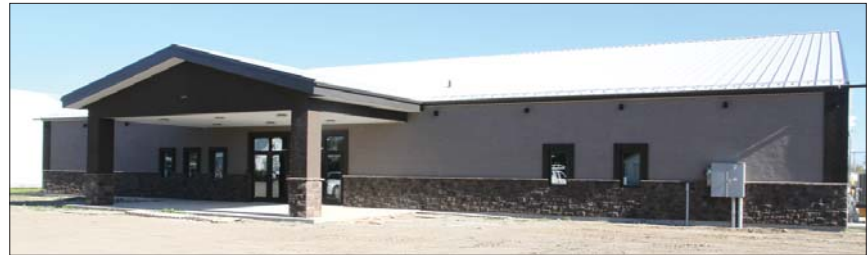
The outside of the Rocanville hall.
