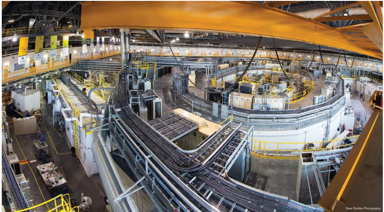
A photo of the Canadian Light Source experimental facility at the University of Saskatchewan from above. See more photos on Page C3.
